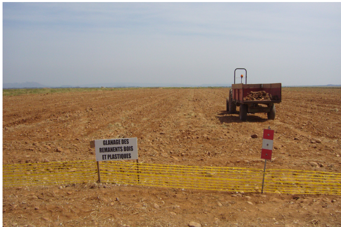
Rehabilitation of the site: recreate the pre-existing topography, soil and vegetation
