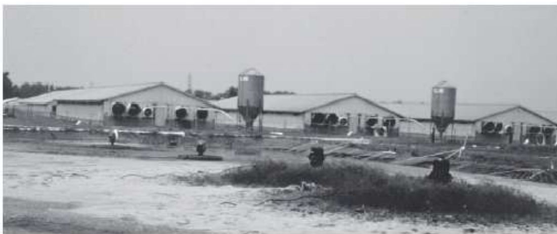
Figure 12: Aerated lagoons treating flushed swine manure.
