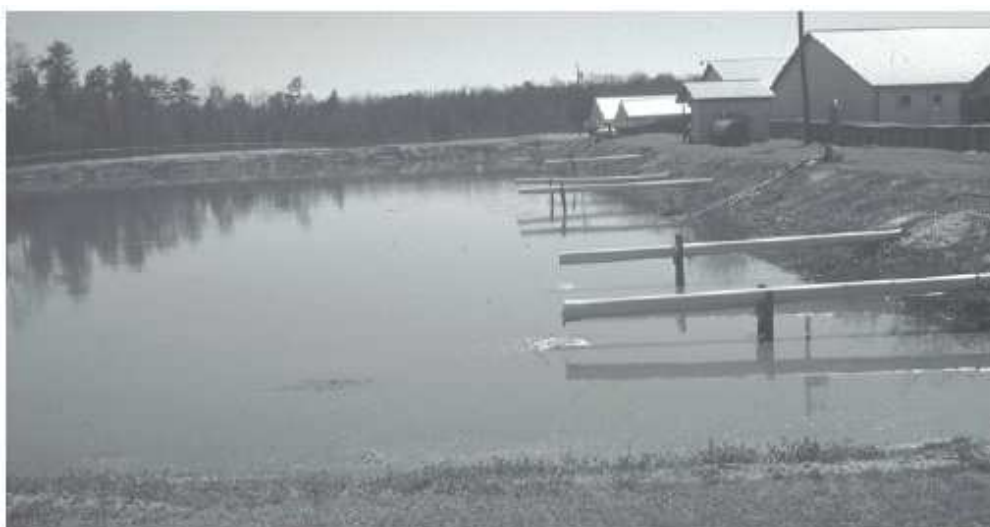
Figure 13: Filling of manure store may degrade the natural surface crust.
